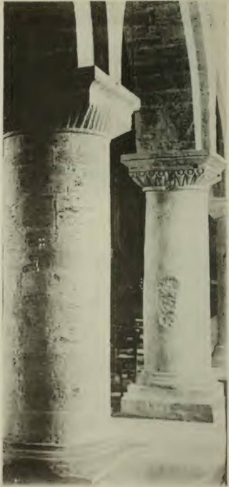
PLATE LVI St. Germain — South West Piers.
